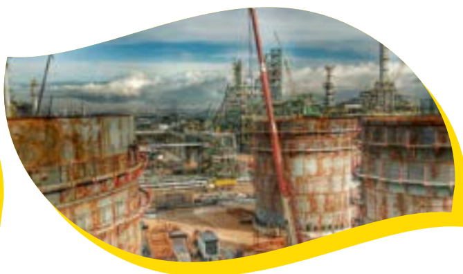
■ Projet: Rehabilitation & Adaptation Project, ALGIERS Refinery, ALGERIA Client: CPECC Année: 2017 - 2018
