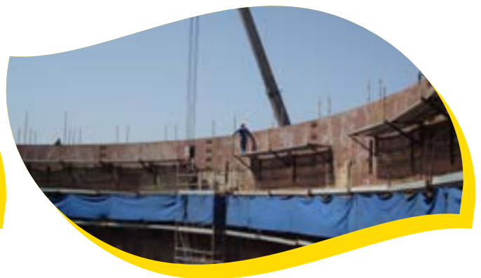
■ Projet: Rehabilitation & Adaptation Project, ALGIERS Refinery, ALGERIA Client: TECHNIP Année: 2014
